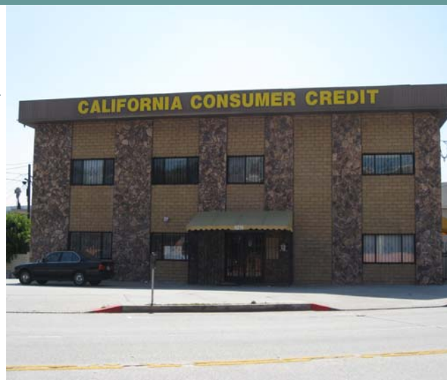
March 26, 2009 - APHCV's new building prior to renovations
